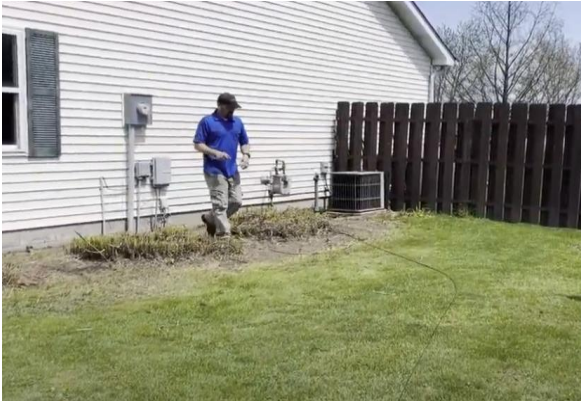
Running the fiber drop to the house
